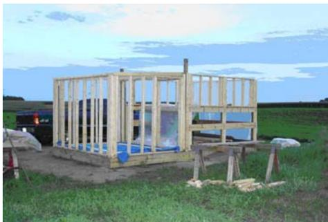
The warm room height at seven feet is set to allow 360 degree rotation of the square dome.
